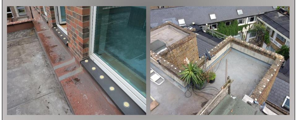
If the ledge is more than 250mm deep, and there is nesting/night roosting in the immediate vicinity of the ledge, two rows of dishes should be applied. Dishes should always be fitted right into the corners of the ledge as birds favour the sheltered corners, and installed in a staggered pattern.
