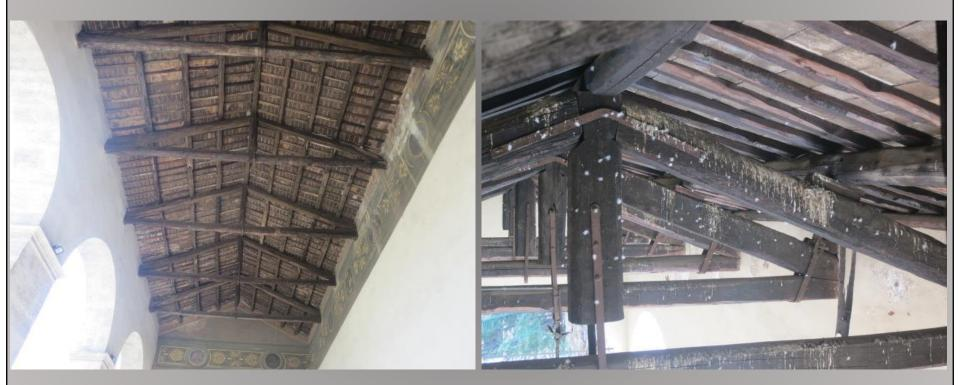
The rafters were first cleaned. Dishes of *Bird Free* were then fitted to the upper parts of the rafters at 200mm centres (below left), and to the lower part of the rafters at 250mm centres (below right).
