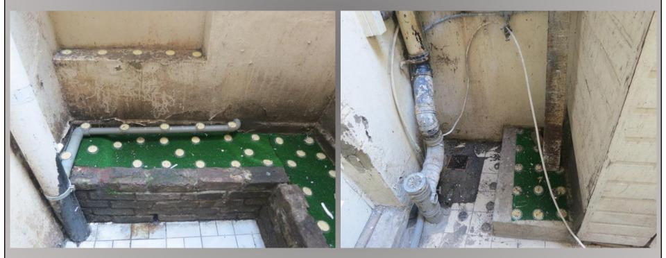
Pigeons nesting in the corner of balconies is a common problem. In this case, the nest must be removed and cleaned using Bird Free Cleaner. Fix four dishes in a square at 150mm centres where the nest was.
